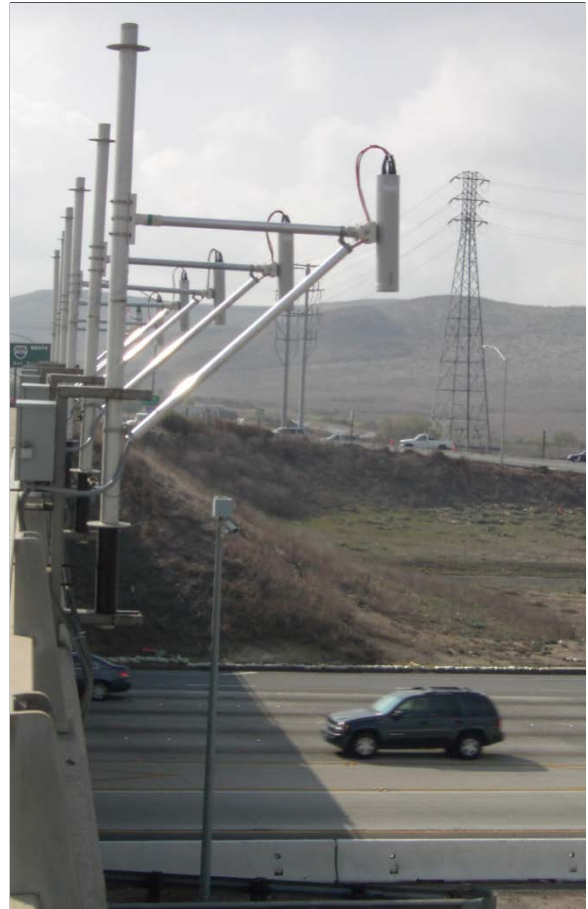
Figure 6.1 Over-lane video cameras and one of two roadside detector masts.
