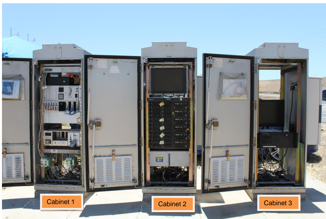
Figure 7.1 V2DVS installed at the Caltrans/Cal Poly Detector Testbed on I-405 near Irvine California. Cabinet 1 contains the detector hardware interfaces including the Type 222 Cardfile. Cabinet 2 contains six V2DVS data acquisition Field Machines, one for each traffic lane. Cabinet 3 contains the V2DVS server.
