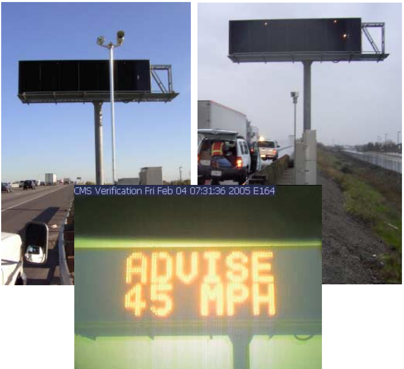
Figure 3.2.4.1. CMS 1, located near County Hospital Road (day on left, ADVISE 45 MPH Message in middle, dusk on right).
